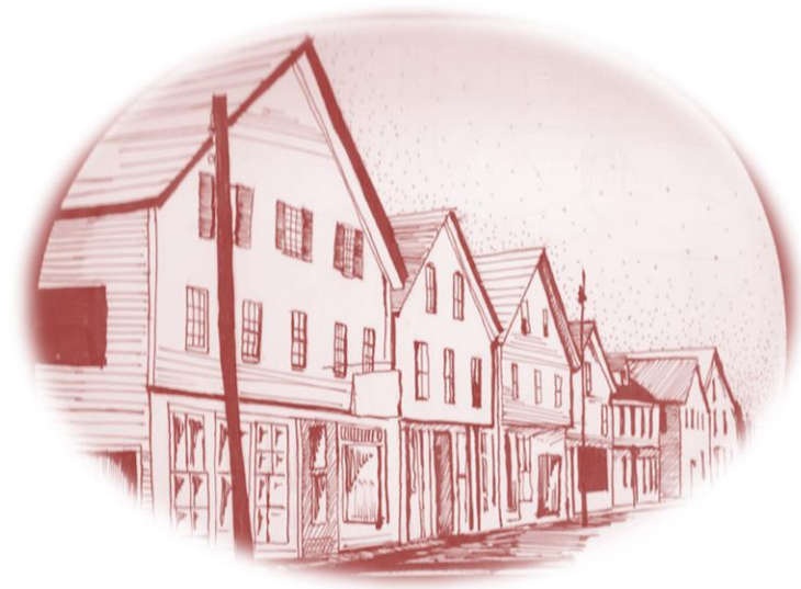
Water Street at King (from early 1980s)
